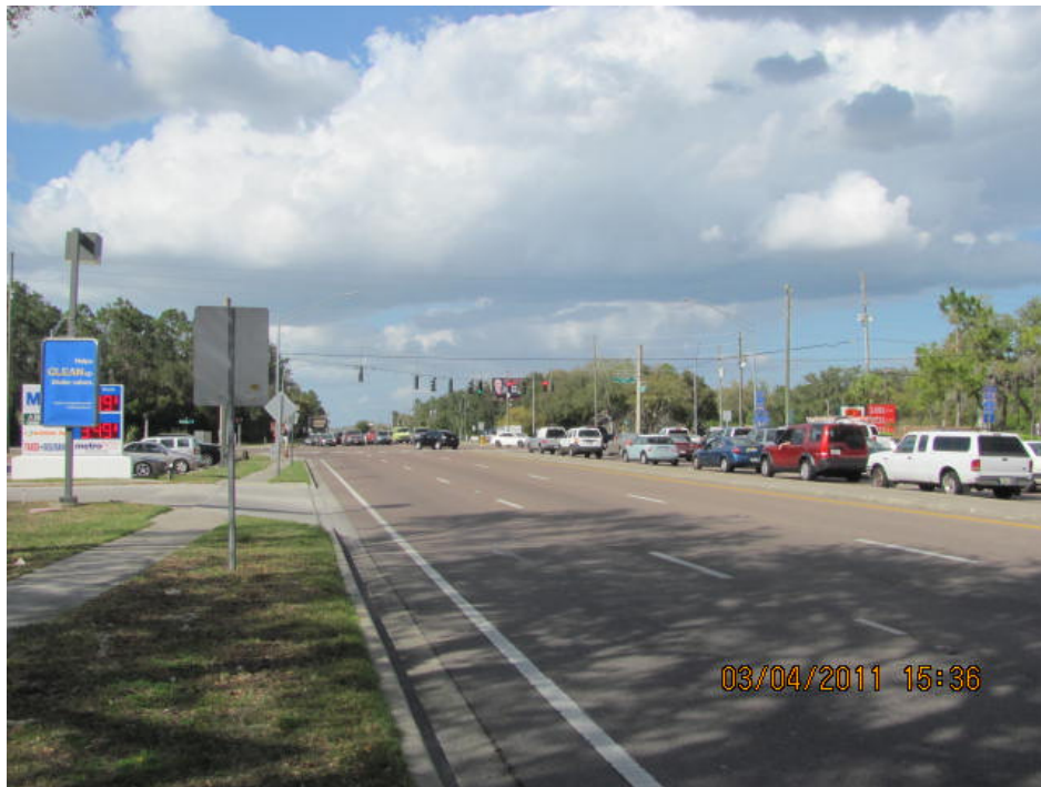
Photograph 8: Looking north along Little Road at the intersection.
