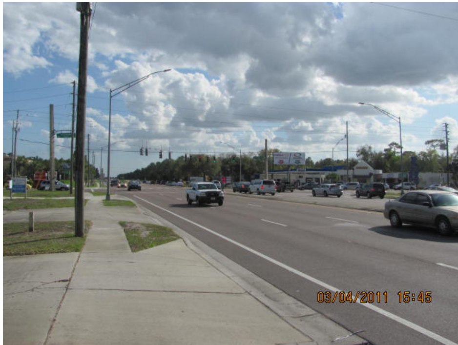
Photograph 5: Looking south along Little Road at the intersection.
