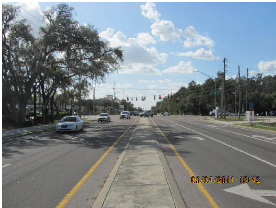
Photograph 6: Looking west along Decubellis Road at the intersection.
