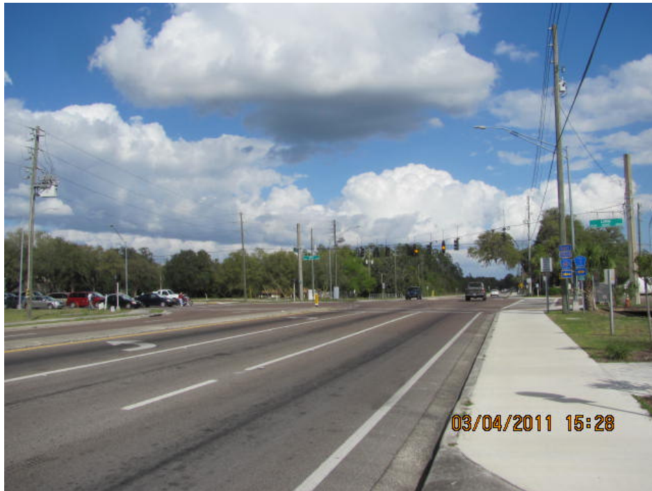
Photograph 3: Looking east along Massachusetts Avenue at the intersection.
