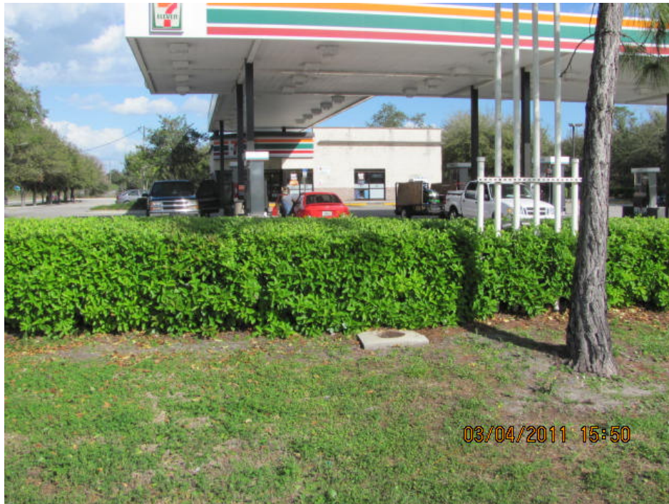
Photograph 15: Monitoring well and vent lines for the 7-Eleven gasoline station.
