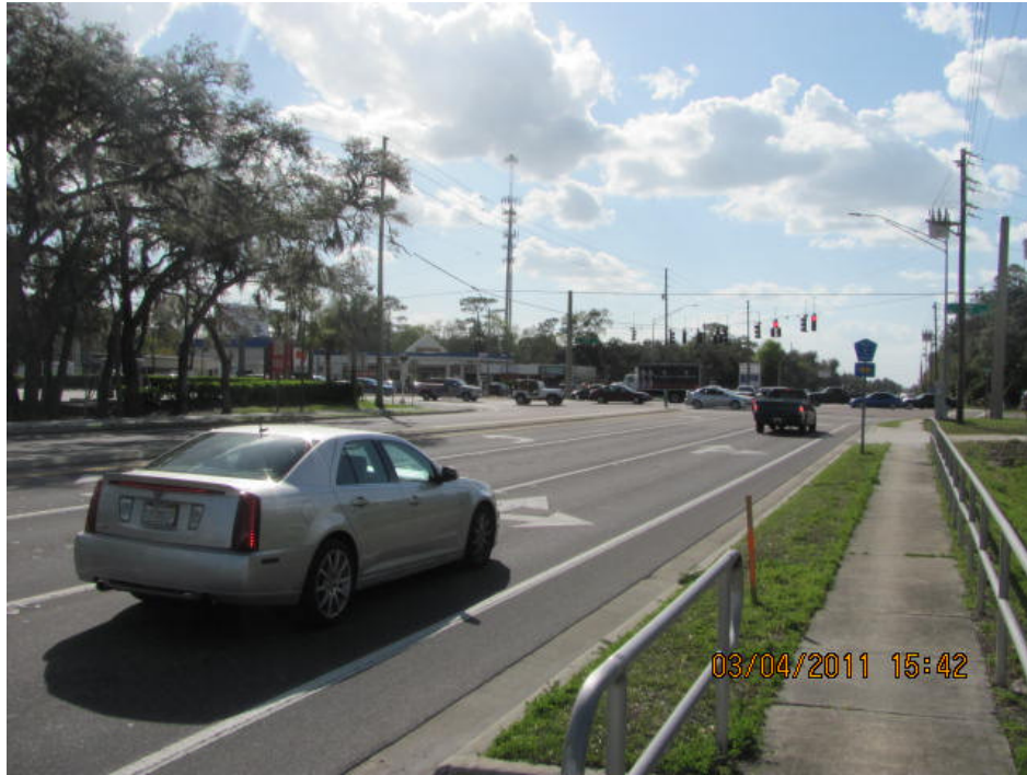
Photograph 7: Looking west along Decubellis Road at the intersection.
