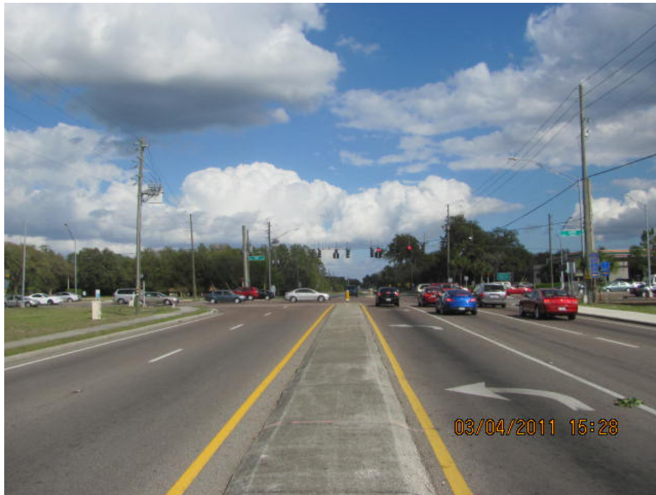
Photograph 2: Looking east along Massachusetts Avenue at the intersection.
