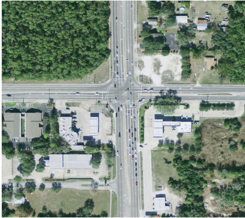
Photograph 1: An aerial view of the intersection (Property).
