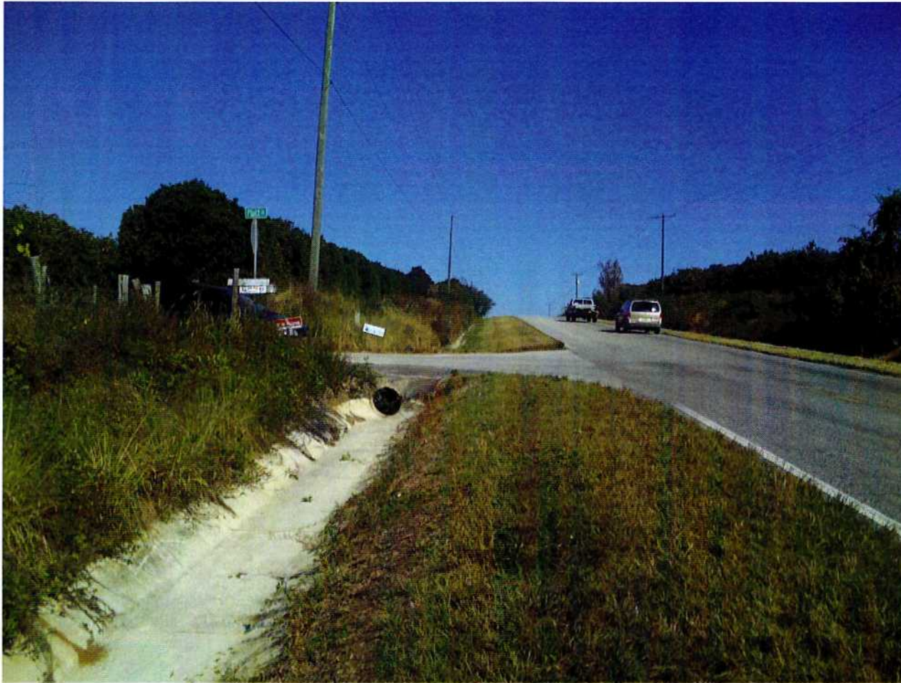
2 – Platt at CR 41. Note the short distance between Platt and top of hill causes potential sight distance problems exacerbated by 55 mph speed limit on CR 41.
