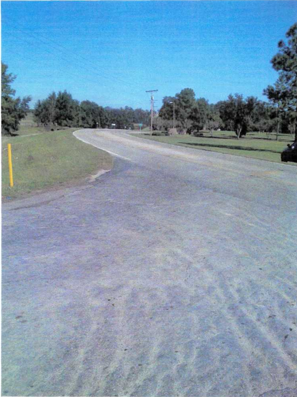
4_ On Ramsey looking at CR 41. Note sight distance issues caused by curve and exacerbated by 55 mph speed limit on CR 41.
